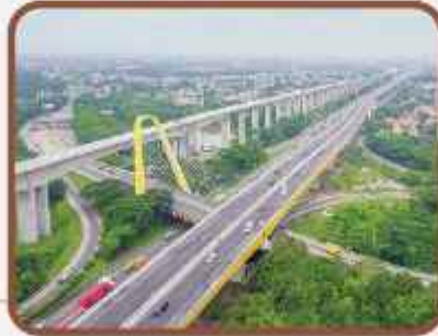
Elevated Toll Ready 100%
